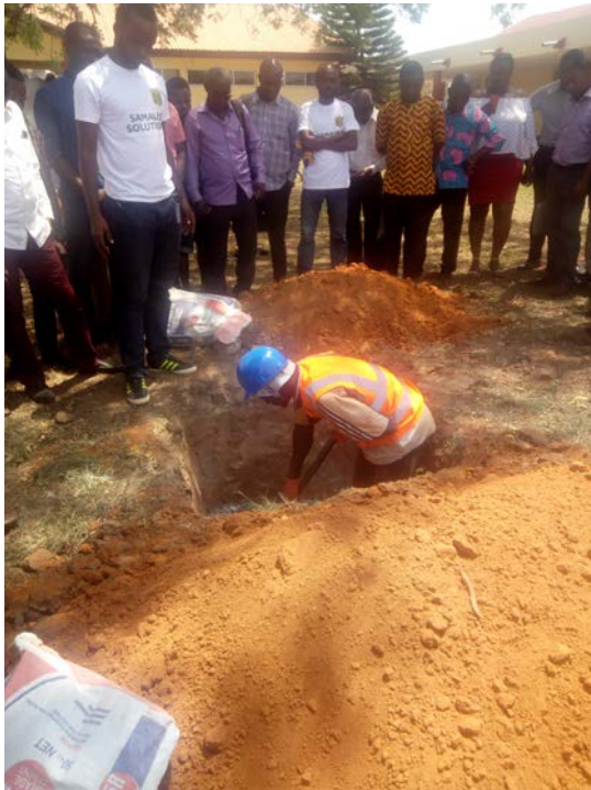
Figure 5: Drain field being dug out
