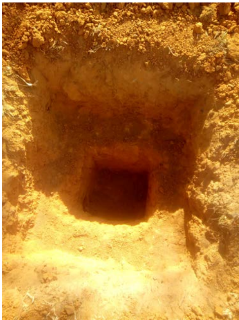
Figure 3: Percolation test hole
