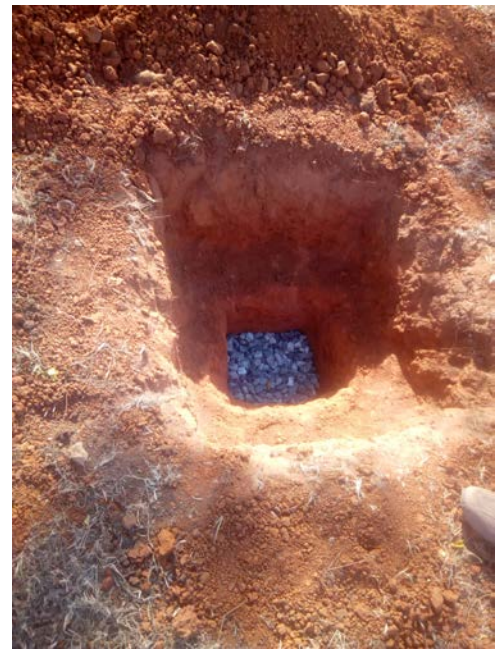
Figure 4: Percolation test hole with gravels
