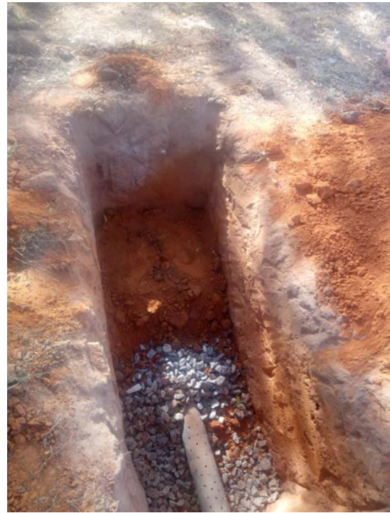
Figure 6: Drain field construction
